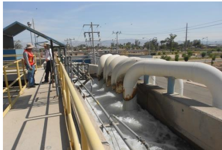
Evaluation of the physical conditions of 234 WWTPs with capacity less than 100L/s
