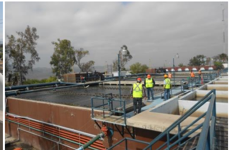
Evaluation of the physical conditions of 234 WWTPs with capacity less than 100L/s
